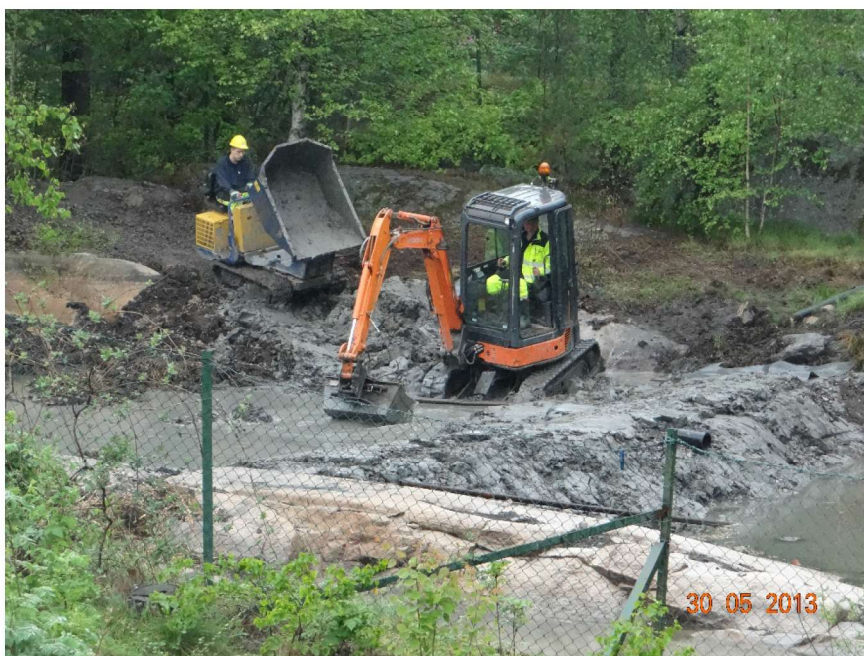
Gravemaskiner lager demning.
